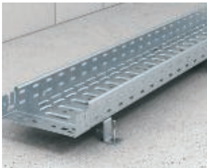
Floor fastening at a distance Installation of a cable tray at a distance using the stand-off bracket DBL. Maximum cable tray width 600 mm.
