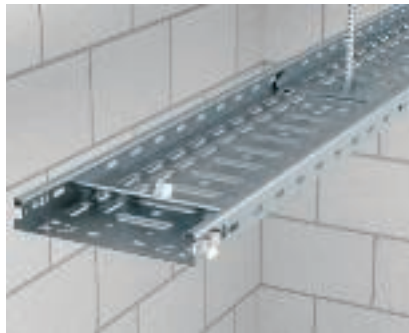
Installation of central hanger MAH 35 Insertion and alignment of the central hanger, MAH 35, in the cable tray.
