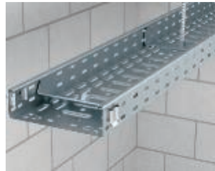
Installation of central suspension MAH 60 Insertion and alignment of the central suspension, MAH 60, in the cable tray.
