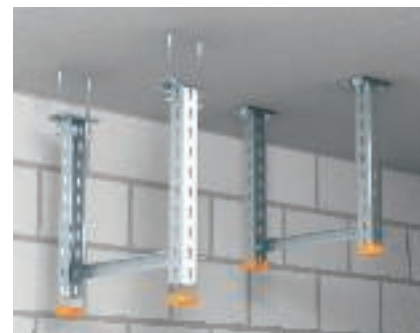
Traverse Installation of U supports US 3 K, US 5 K and US 7 K under the ceiling using anchor bolts, FAZ II, and use of a trapeze, consisting of U profile US 3, US 5 or US 7.
